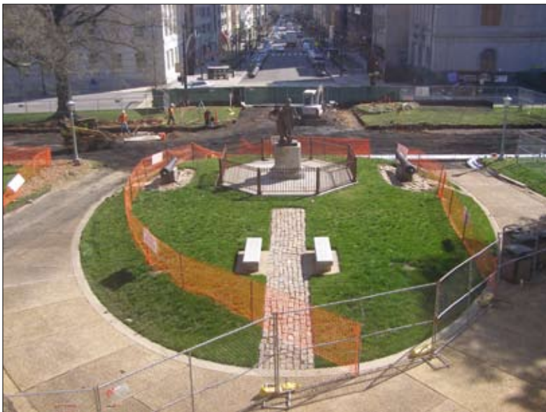
Above: This photograph, taken March 20, 2009, shows how the south plaza looked after crews removed the old pavement and prepared to pour the new concrete.
